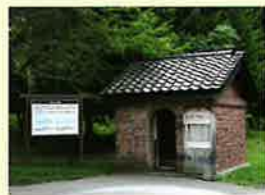
Brickwork Punishment Chamber
